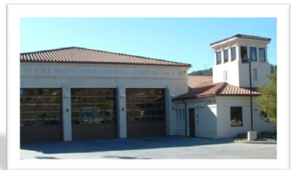
Station 65 5 Bolling Drive
