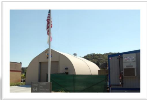
Station 64 105 Roblar Drive
