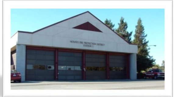
Station 61 7025 Redwood Blvd
