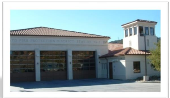
Station 65 5 Bolling Drive
