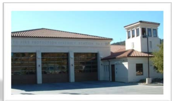
Station 65 5 Bolling Drive
